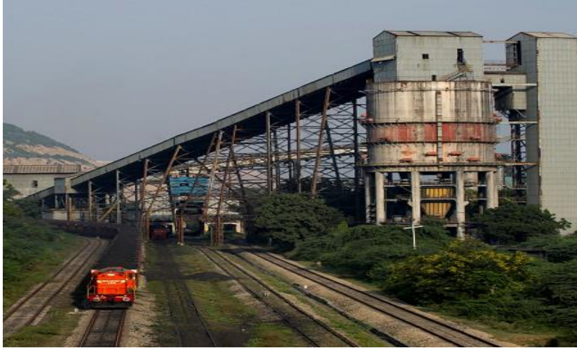
Mechanised evacuation of coal from the pithead to the dispatch point
