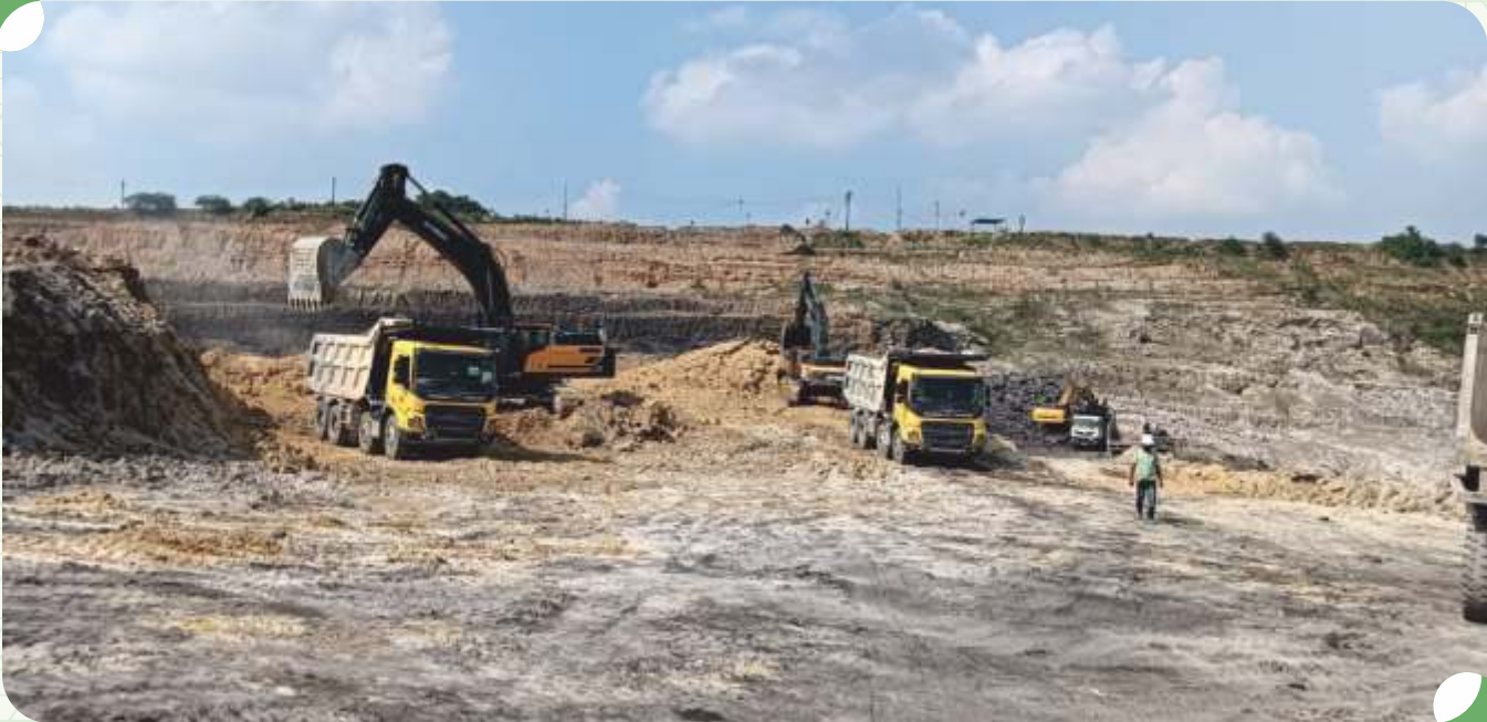
■ Overburden Removal work in progress at one of Opencast Mine, WCL.
