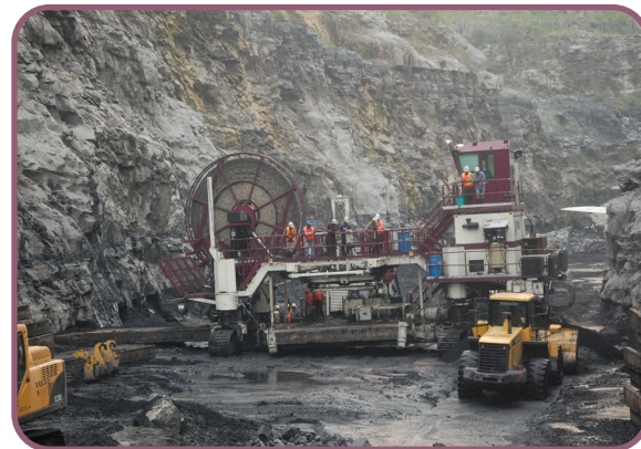
Highwall Operation at Sharda Mine, Sohagpur Area
