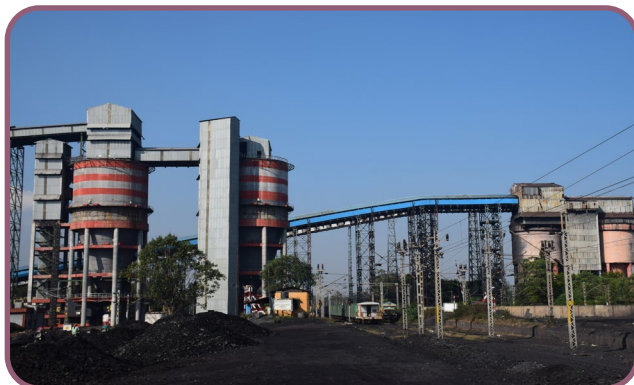
Rapid Loading System-SILO at Gevra Area
