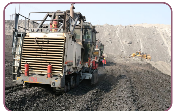
Surface Miner in Operation at Gevra OC
