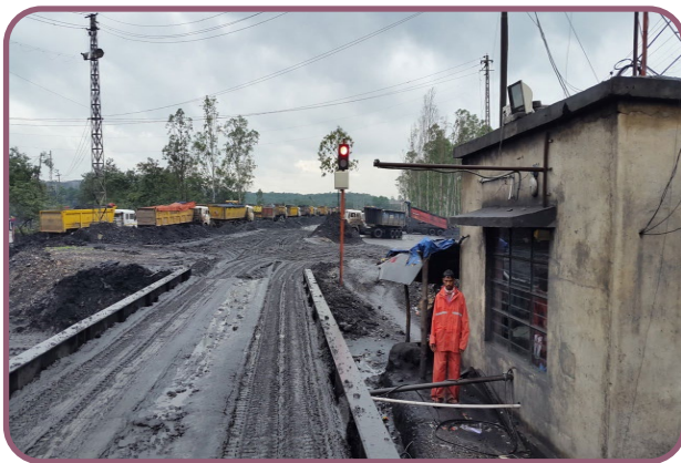
Red light indicates absence of Vehicle in WB or incorrect position of vehicle at WB during weighing.
