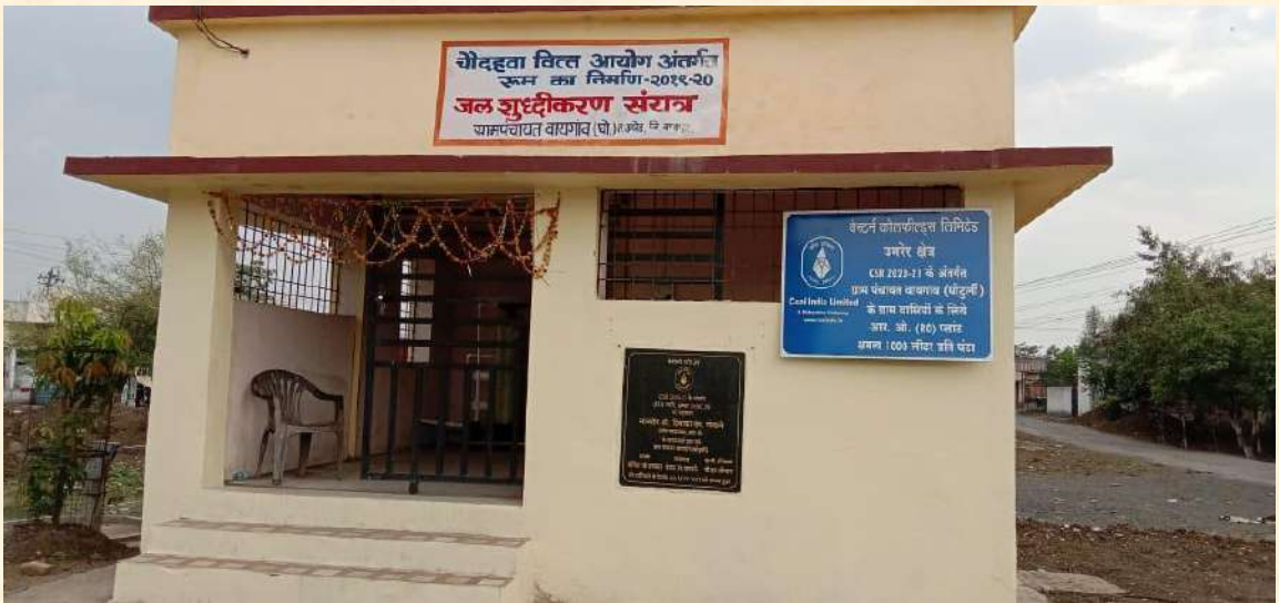
Fig. 68 - Water Purification Plant by Umrer Area, WCL
