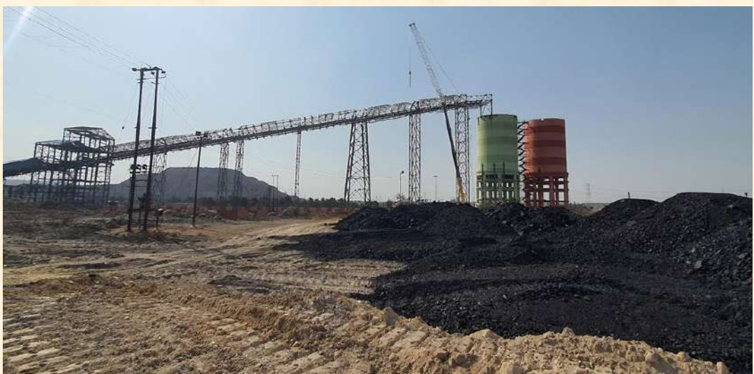
Fig. 15 - Silo under construction in Sonpur Bazari OC of ECL
