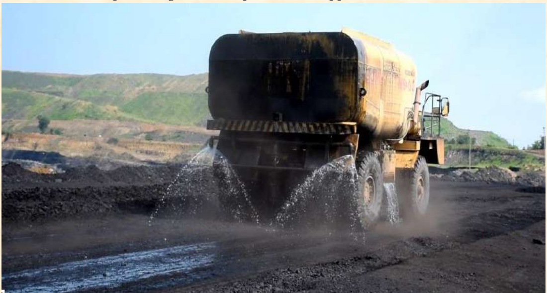
Fig. 48 - Mobile Sprinklers in operation for suppression of dust
