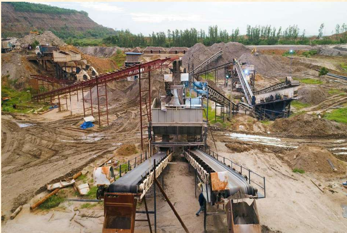
Fig. 50 - OB to sand plant in WCL
