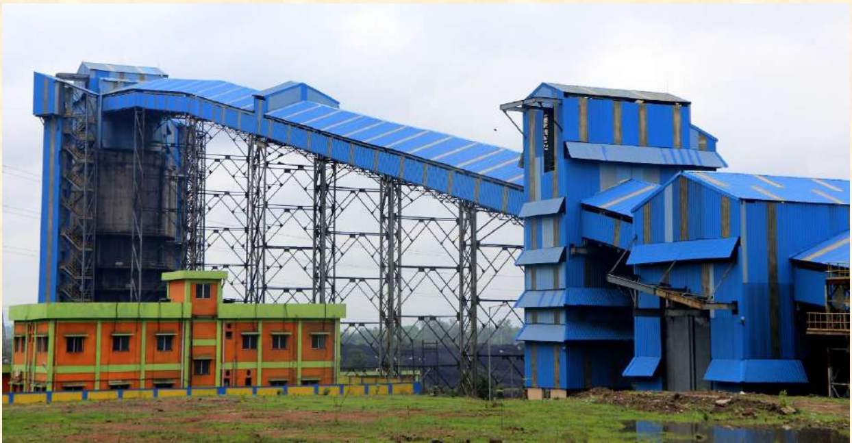
Fig. 17 - Silo in Lingaraj OCP of MCL
