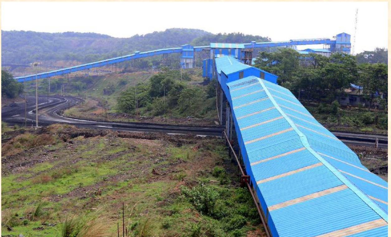
Fig. 17 - Silo in Operation at Lingaraj OCP of MCL
