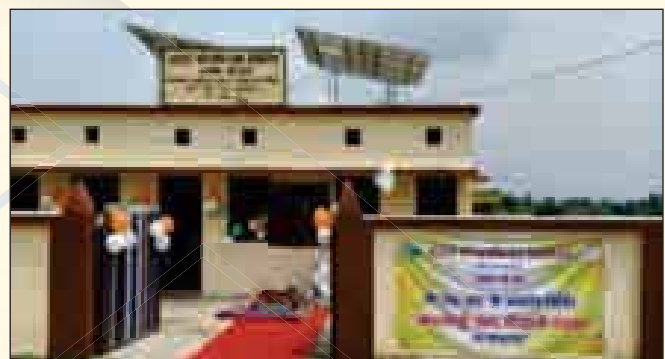
Image 7 : Construction of Govt. Girls high school at Panjreh, Singrauli and Anganwadi building at Gondwali Gram Panchayat.
