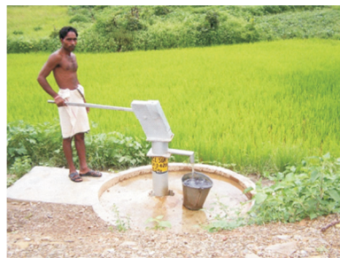
Hand pump installed by NCL
