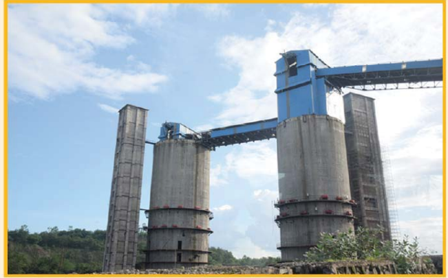
SILO under construction at Bharatpur Area
