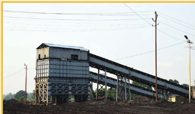
Coal Handling Plant Lingaraj
