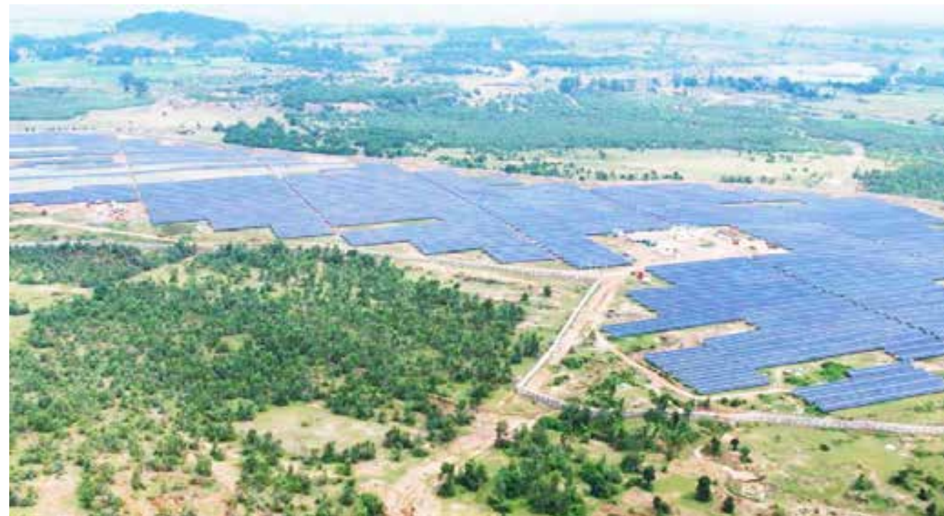
► 20 MW Solar Power Plant at SECL Bhatgaon Area
