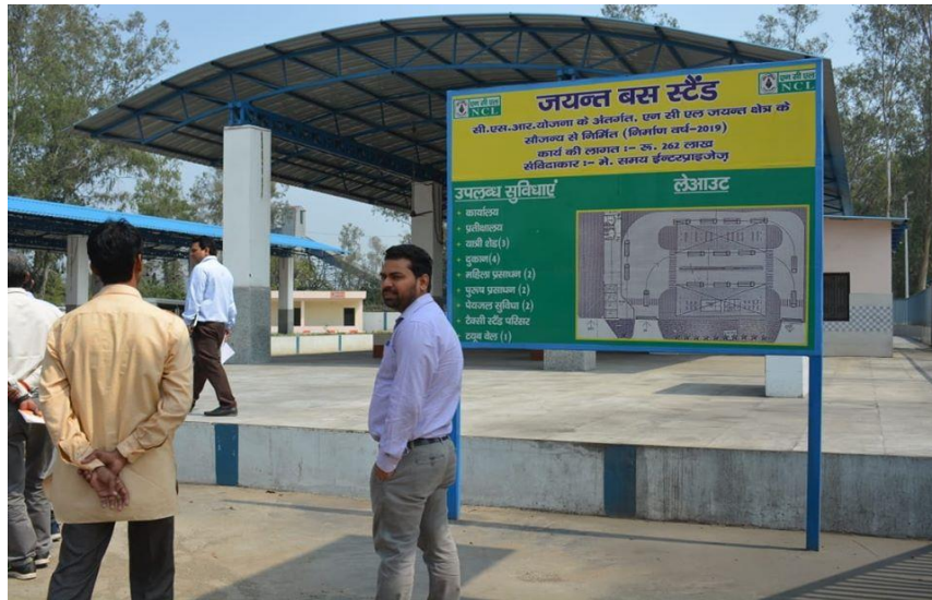
Fig. 87 - Construction of new bus stand at Jayant in Madhya Pradesh, Northern Coalfields Ltd
