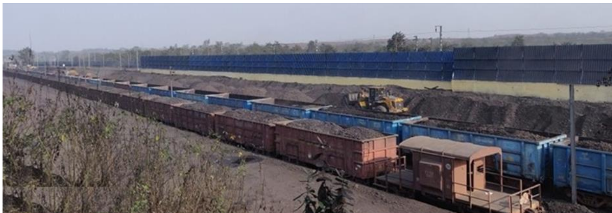
Fig. 48 - Vertical wind barrier to arrest dust propagation in MCL
