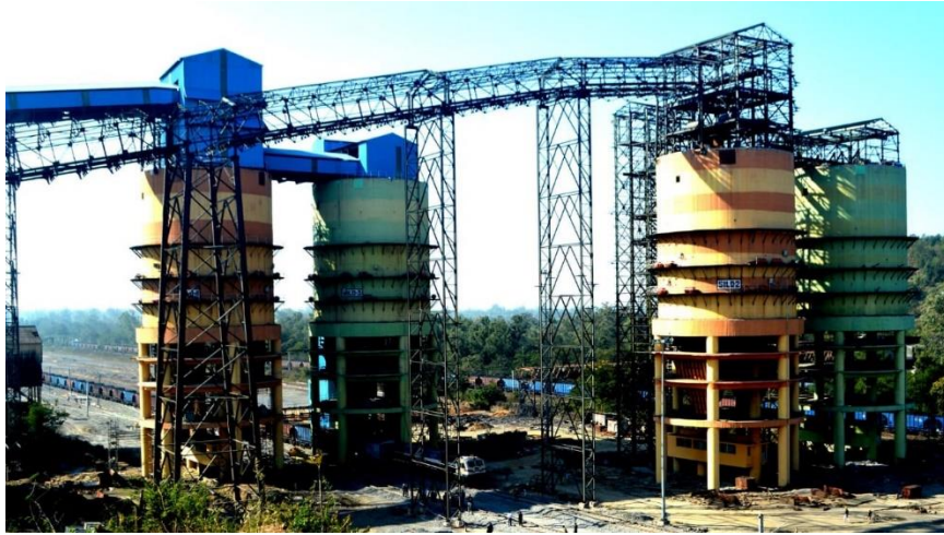
Mechanised evacuation of coal from the pithead to the dispatch point
