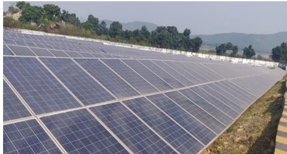
Ground mounted solar panels at MCL
