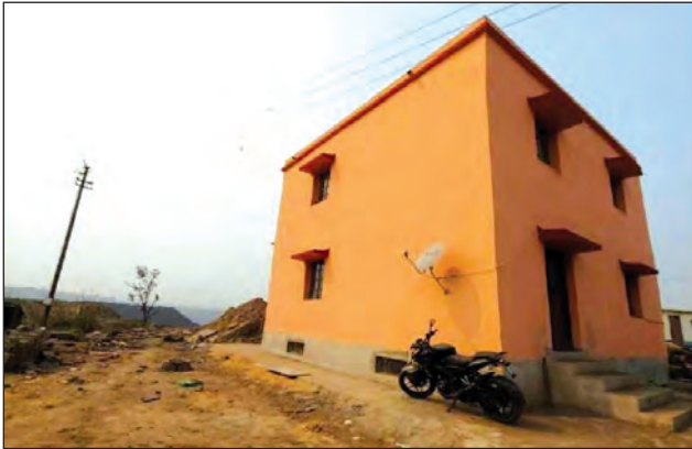
Prototype Building constructed at Jagannath Area, MCL for S&T project titled constructing structures on backfilled opencast coal mining- an attempt to suggest viable methodologies
