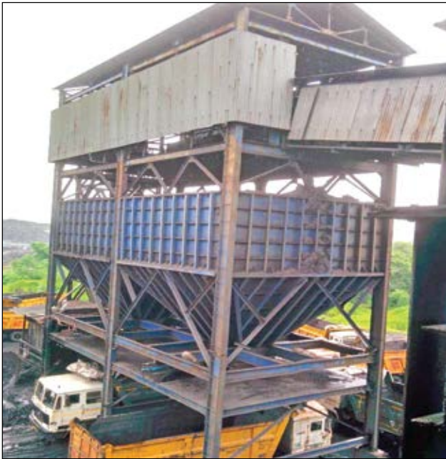
Figure 1 : Site Photo for Truck Receiving Hopper at Mungoli CHP, WCL.
