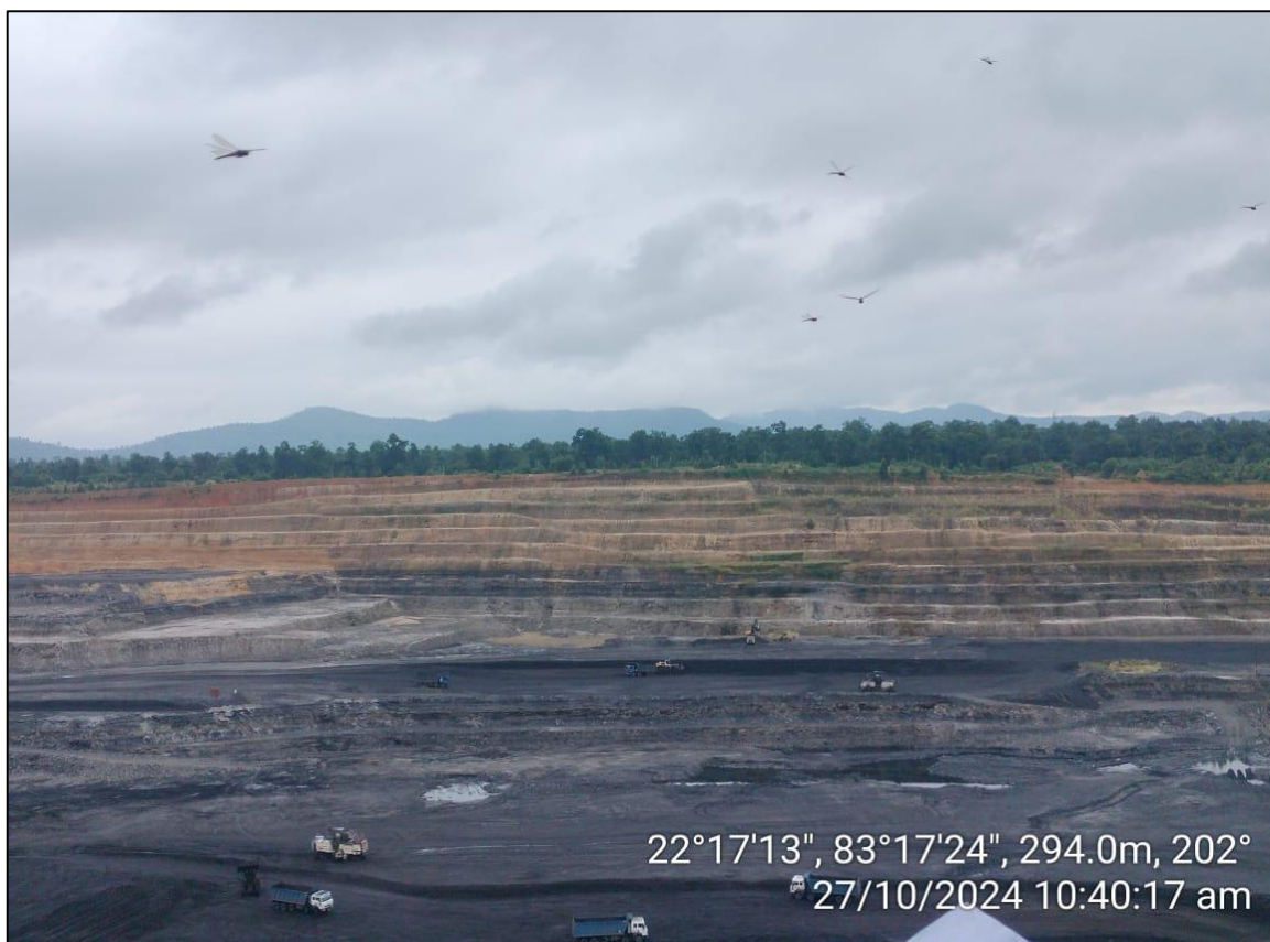
Photo 6.13: Overview of Jampali Opencast Project
