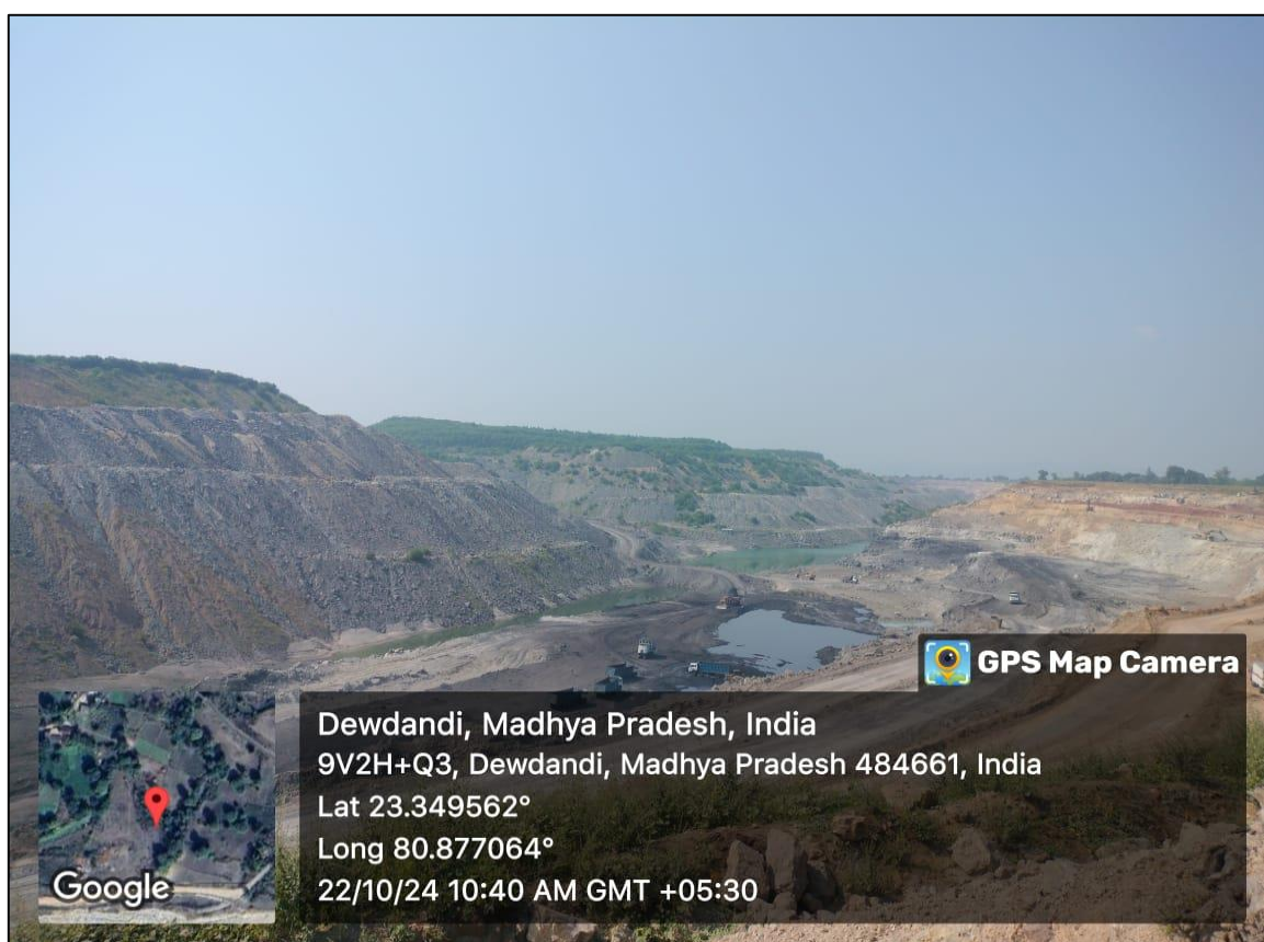
Photo 6.22: Overview of Kanchan Opencast Project
