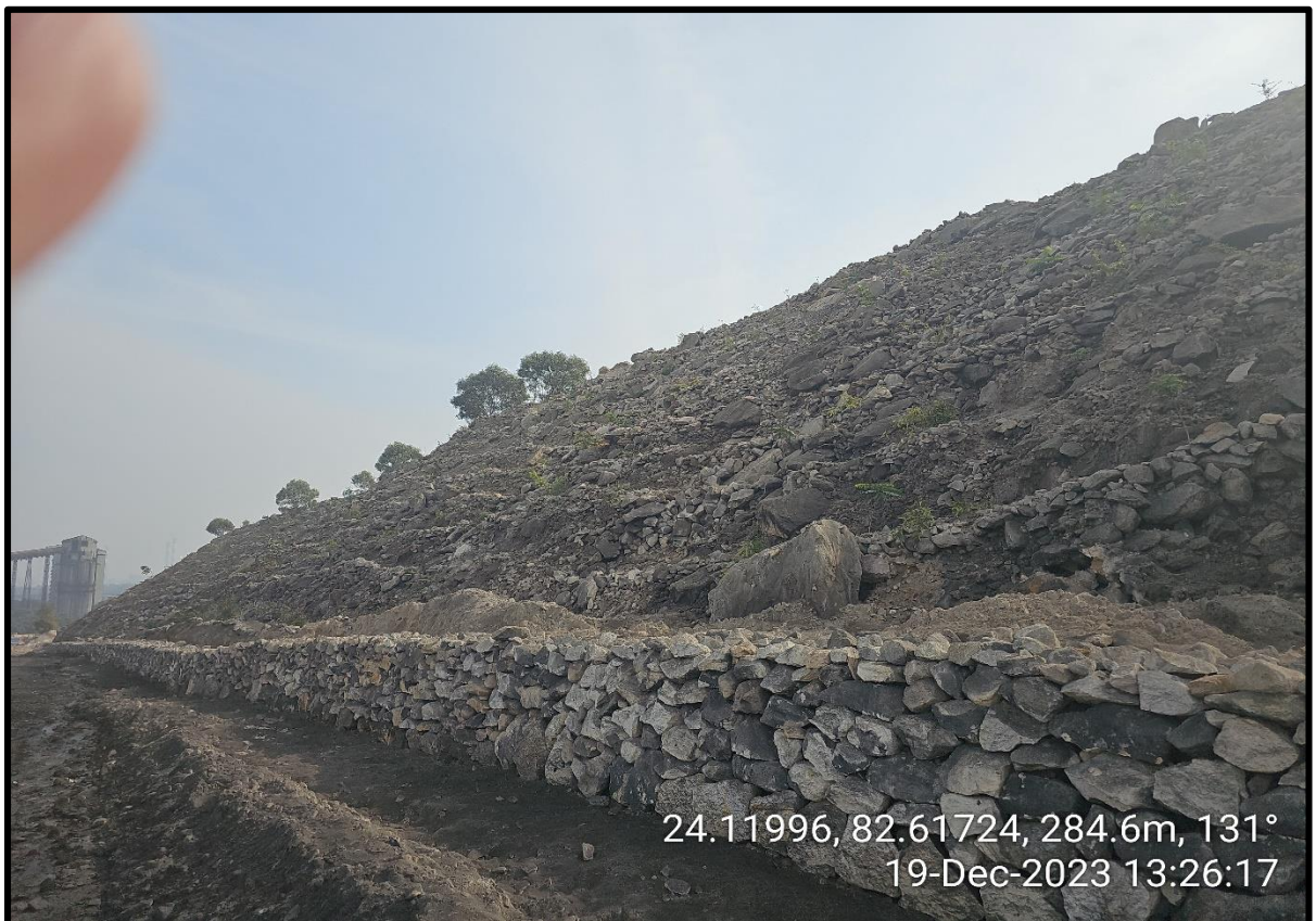
Photograph 7.2: Nigahi OCP- Plantation growing on the Backfill
