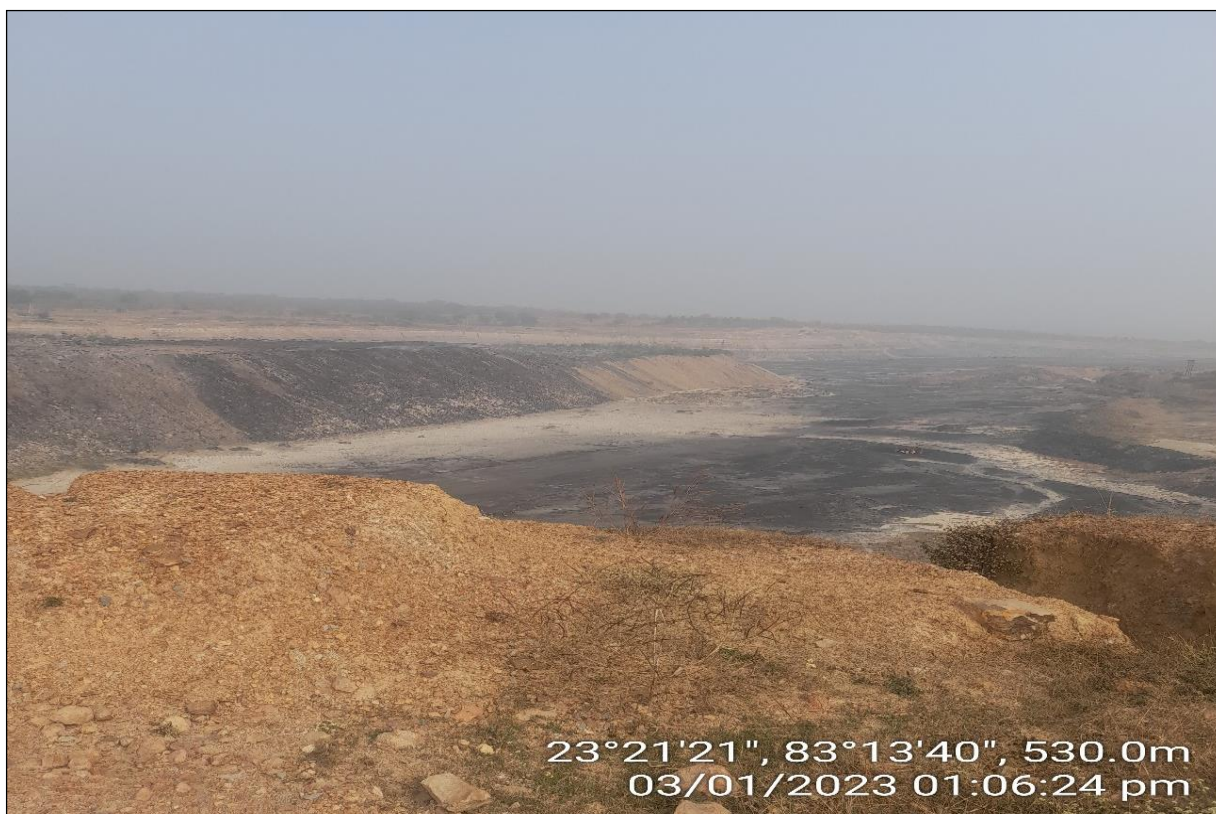
Photograph – 6.23: Overview of Mahan- II Opencast Project
