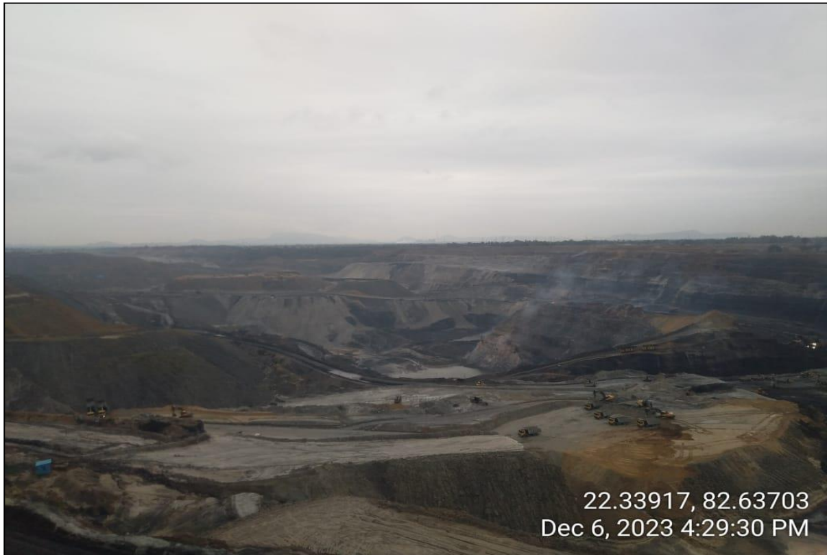
Photograph – 6.5: Overview of Kusmunda Opencast Project
