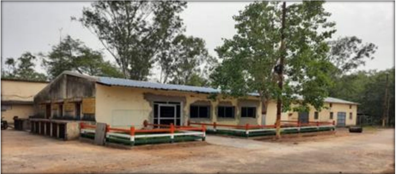
Fig. - Exterior View of under-construction museum
