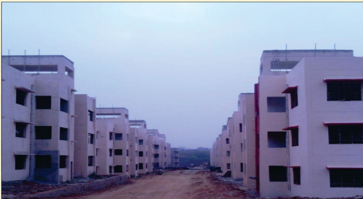
Miner's quarter completed at Lodna
