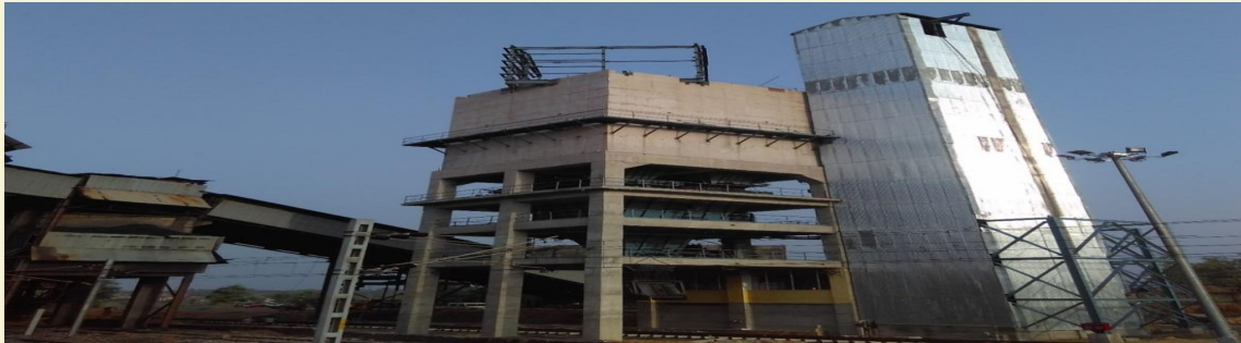
5.0 Mtpa MADHUBAND NLW WASHERY UNDER CONSTRUCTION
