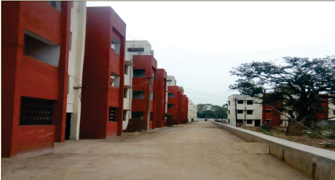
Miner's quarter completed at CV Area
