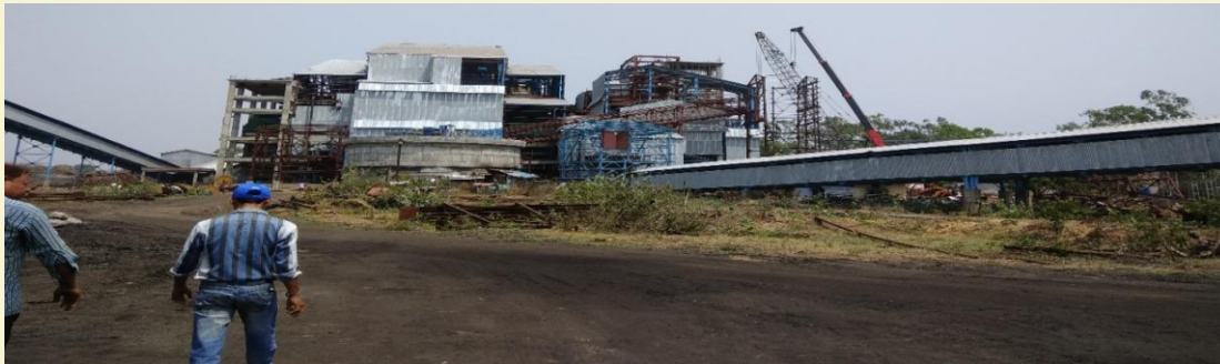
5.0 Mtpa PATHERDIH NLW WASHERY UNDER CONSTRUCTION
