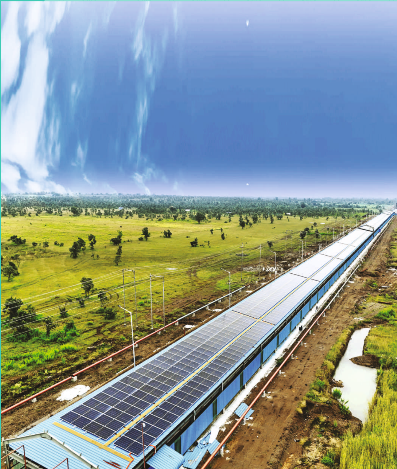
3 MW Roof Top Solar Power Plant at CHP-SILO, Umrer Area.
