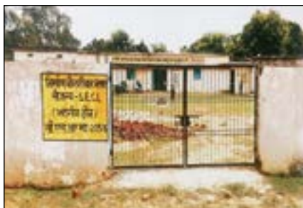
Boundary wall at Belpara Primary School Building of Karondha village
