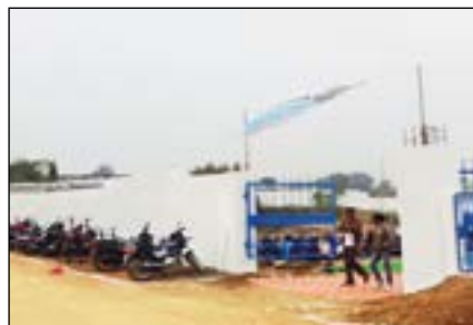
Construction of Boundary wall at Eklavya Banvasi Balchhatravas, Manendragarh, Dist. Korea
