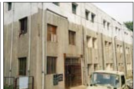
Construction of 20 bed ICU unit along with financial assistance for ICU Equipments at District Hospital Ambikapur (Surguja)
