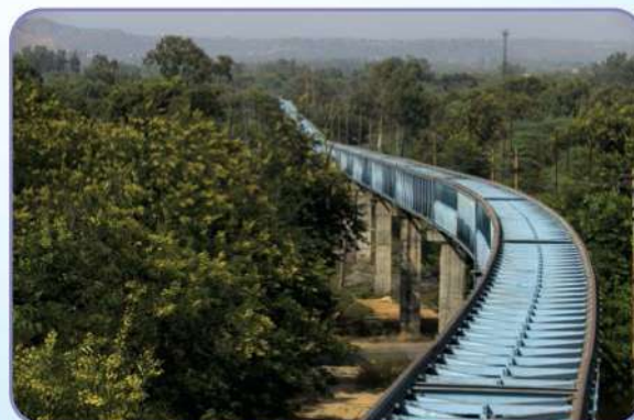
Environment friendly Pipe conveyor system
