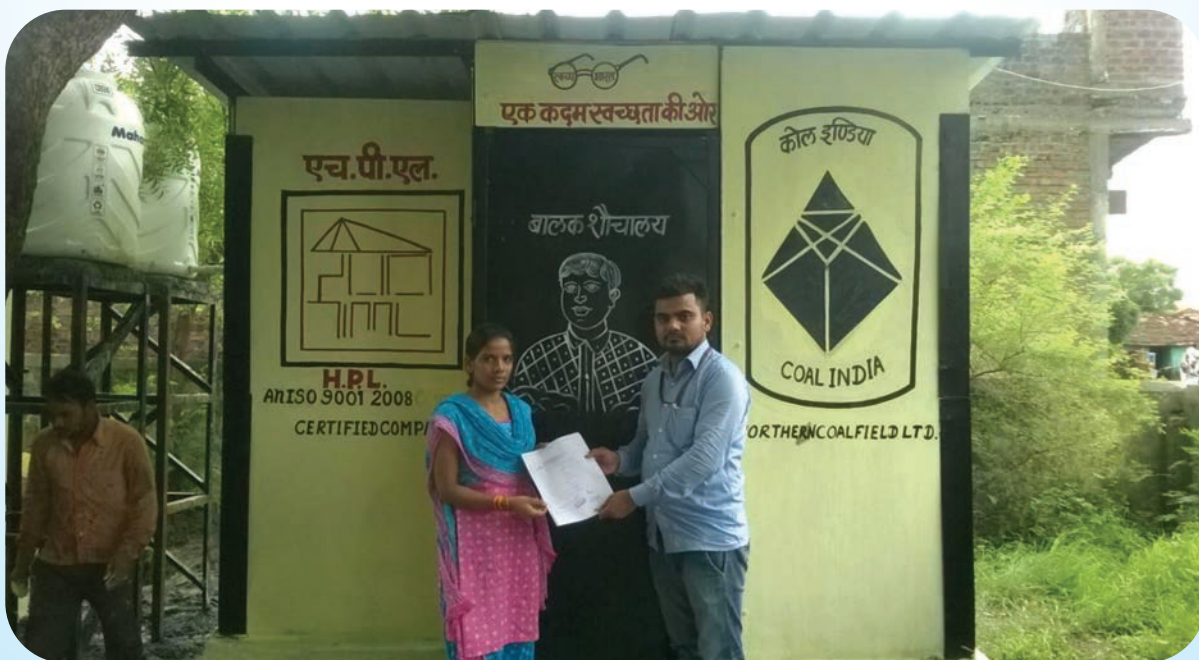
Toilet constructed under Swachh Bharat Abhiyan by NCL
