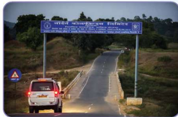
15 Km road from Singrauli Rly station to Parsohar constructed by NCL under CSR
