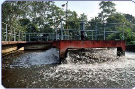
STP at Amlorhi Project of NCL
